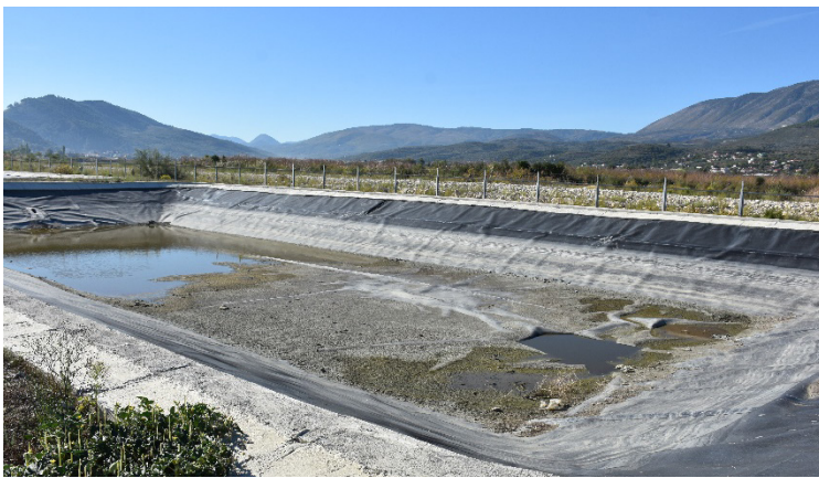
A new deposit site in Berat municipality ensures that gas emissions are controlled and leakages do not flow into the river Osum.
