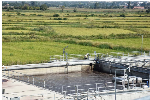
Kocani Waste Water Treatment Plant. Photo: Ljubinka Ajtovska
