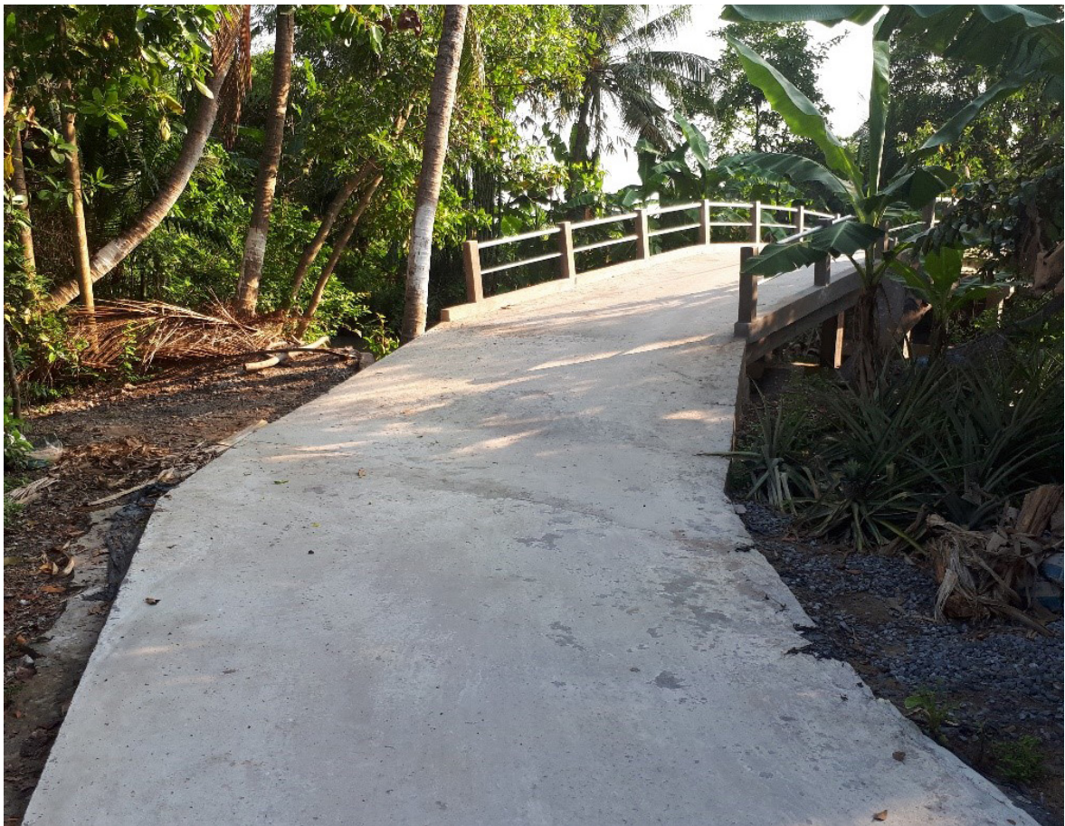
Figure 25: Recently completed bridge with flush transition to the connecting road. No land subsidence visible yet.
