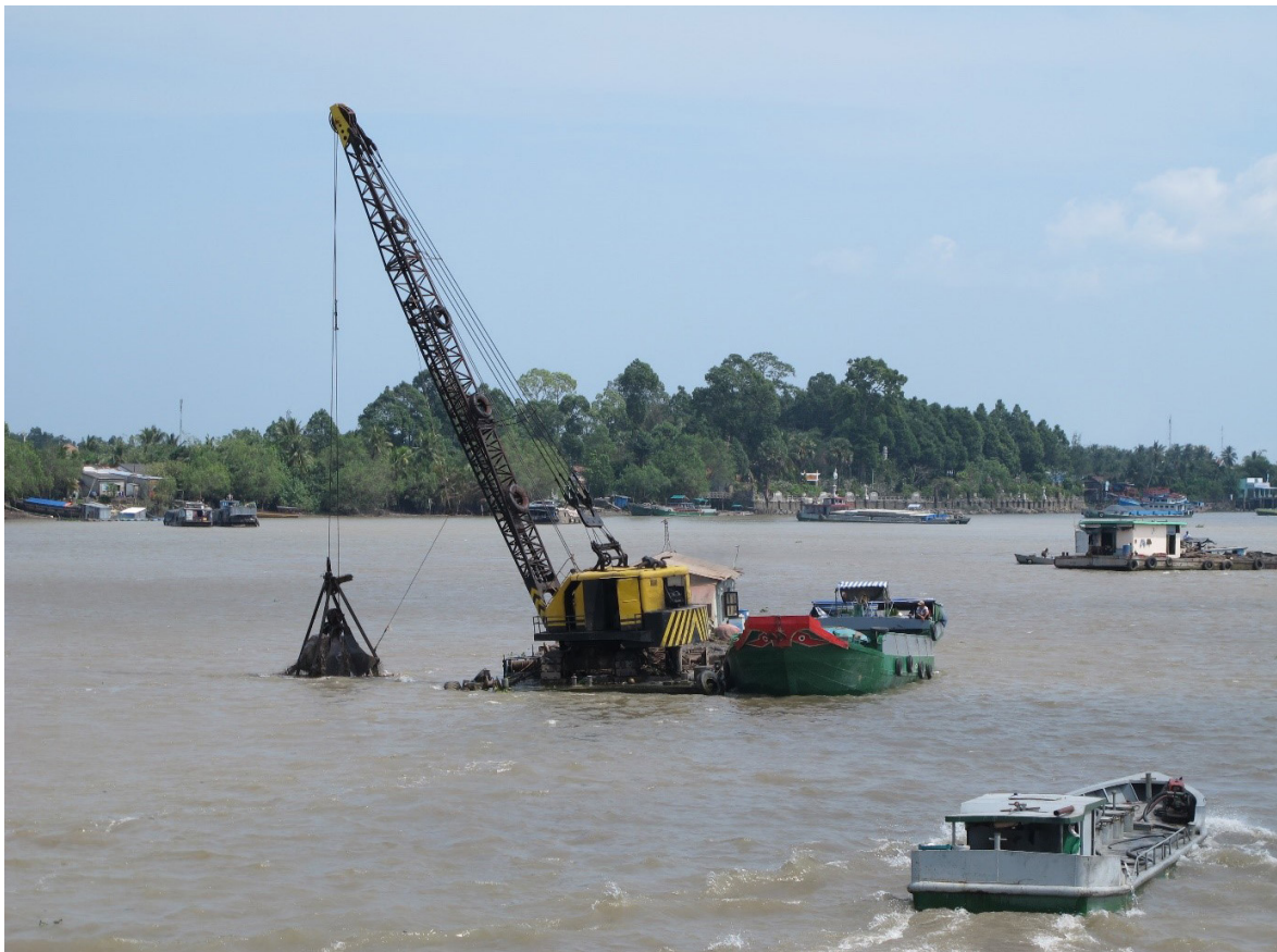
Figure 36: Sand mining in the Mekong River
