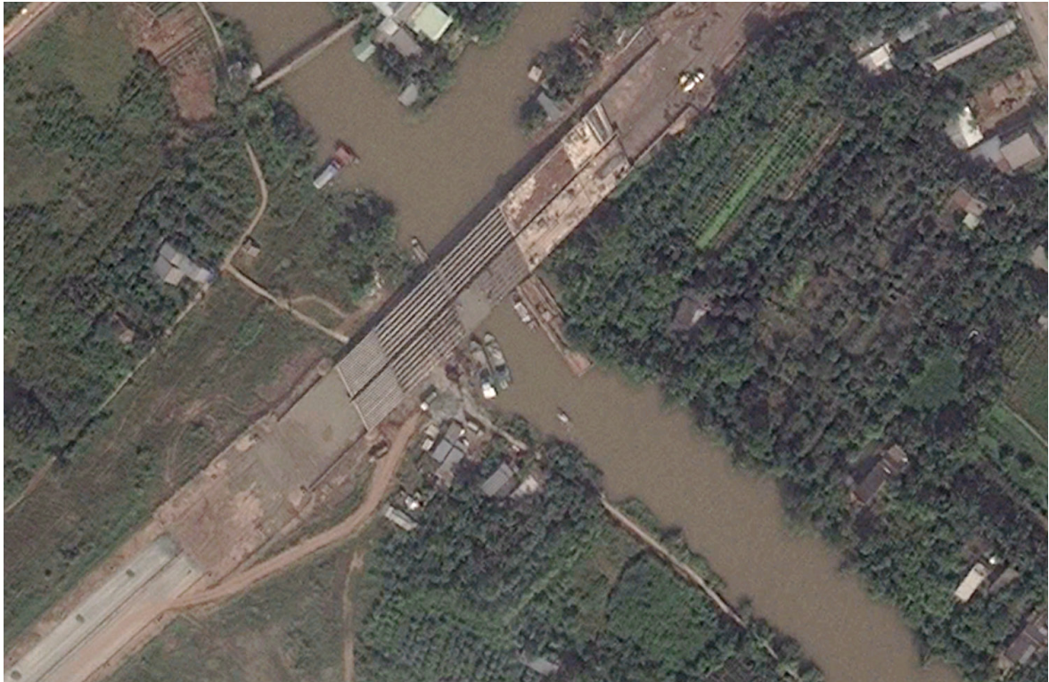
Figure 26: Google Earth image of Cau Cai Son Bridge from 08.12.2009. Ten years later the bridge is approx. 35 cm higher than the connecting road. On average the road sank 3.5 cm/year relative to the bridge.
