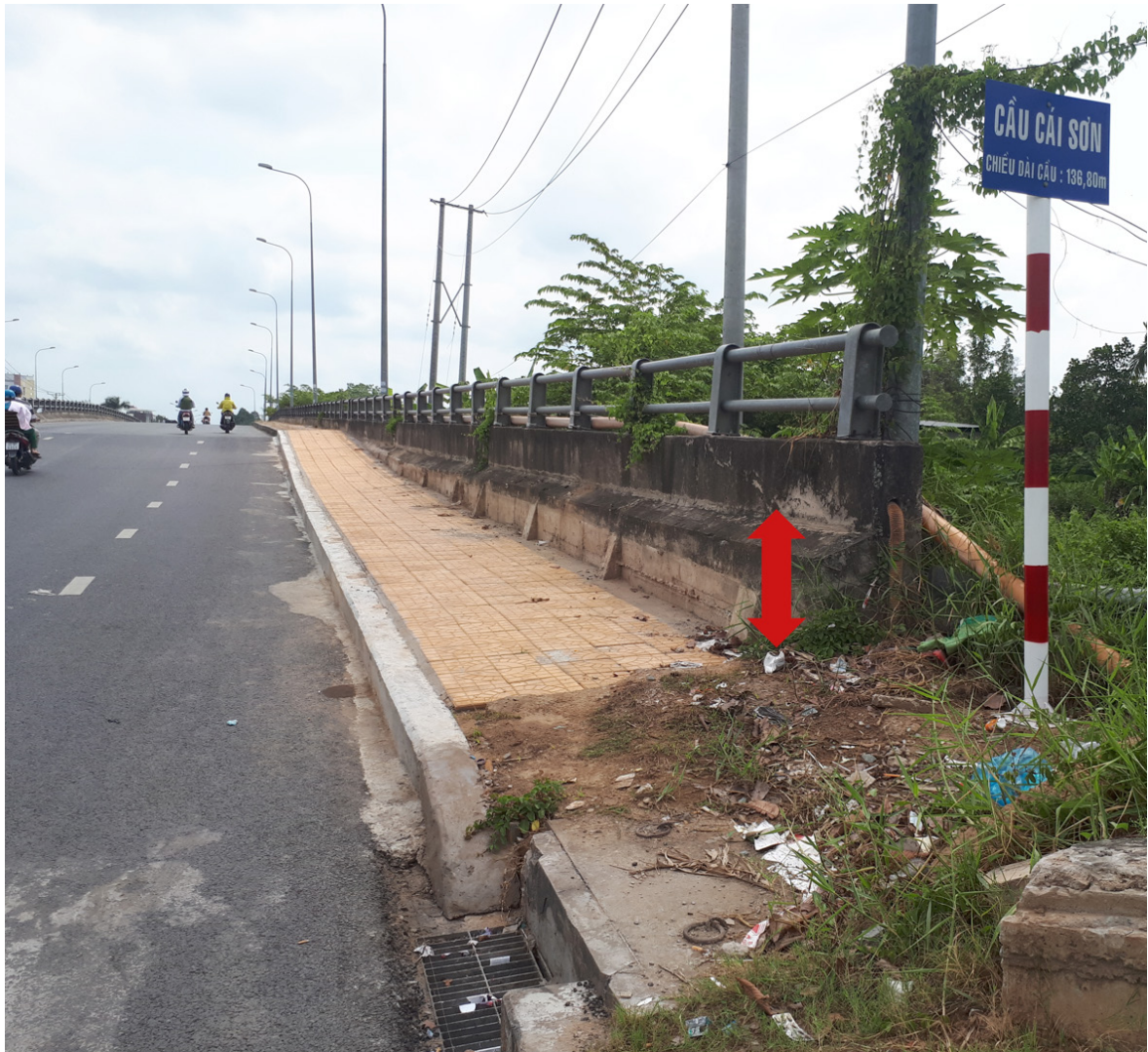
Figure 28: Image of Cau Cai Son Bridge from early 2019
