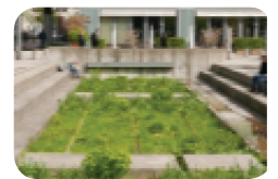
Rain gardens or bio-retention systems
