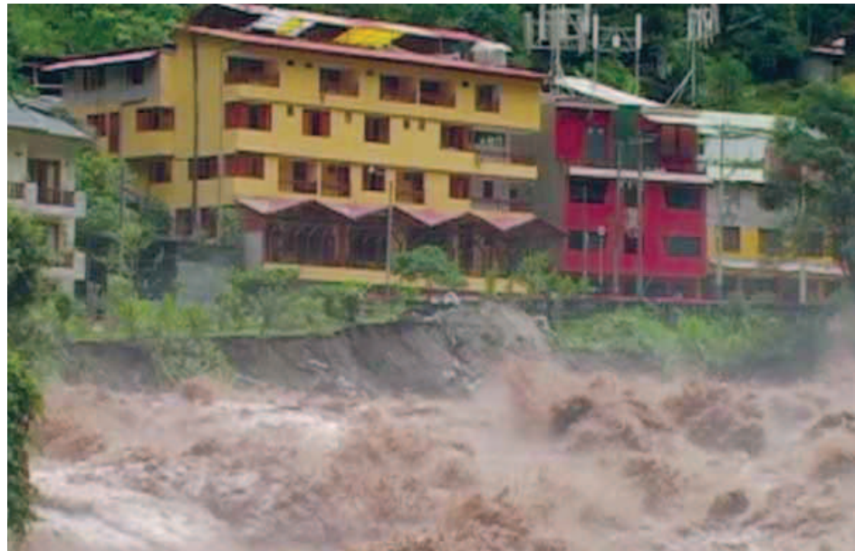
High-cost tourism infrastructure exposed to a mountain torrent Location: Aguas Calientes near Cusco, Perú. Photo credit: La Republica, February 2010
