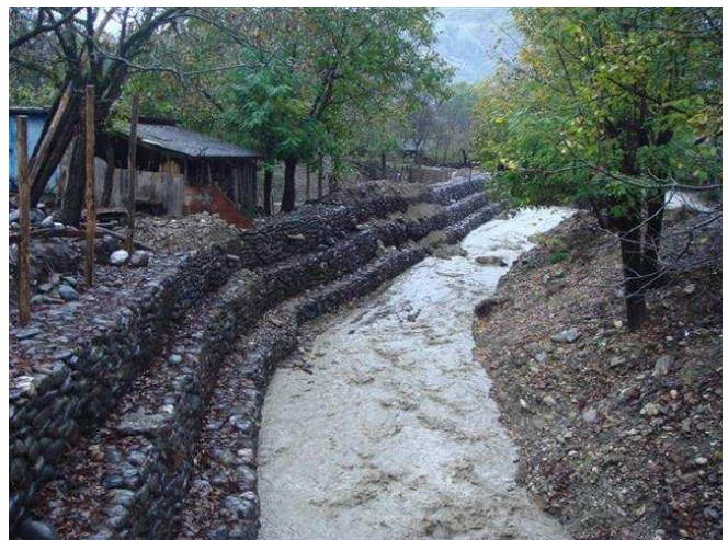
Gabions as an example of local risk reduction measure to prevent river erosion and flooding.
