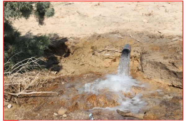
Pumping water to the wetland
