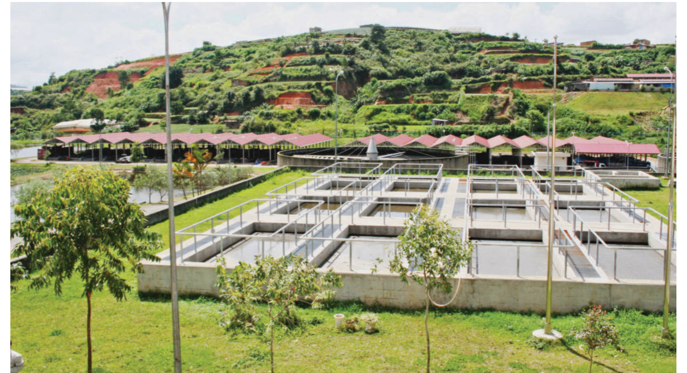
Da Lat Wastewater Treatment Plant, Lam Dong Province
