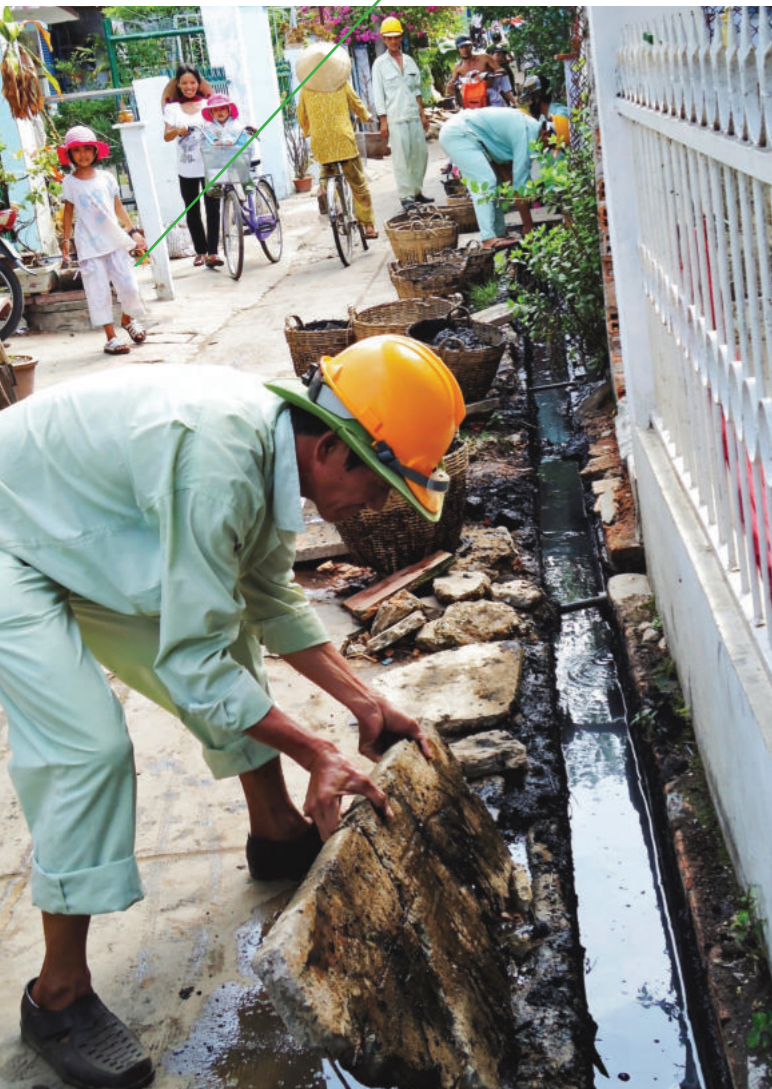
Dredging the canals
