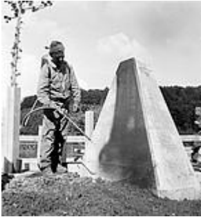
Construction of anti-tank obstacles in the 1940s. They were also nicknamed "Toblerone" due to their resemblance to the famous Swiss chocolate bar. © Theo Frey/Swiss Federal Archive Bern
