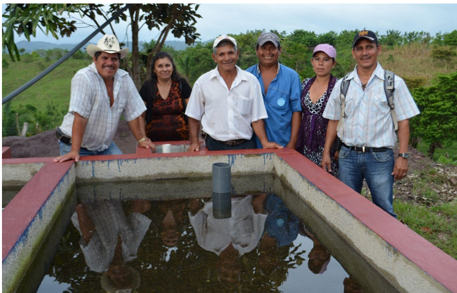
The pride of access to drinking water: The water committee of the village "Walter Calderon" visits the newly installed filter system
