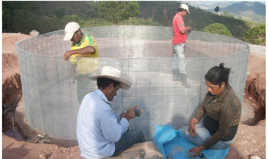
The drinking-water system is built in teamwork by the local community
