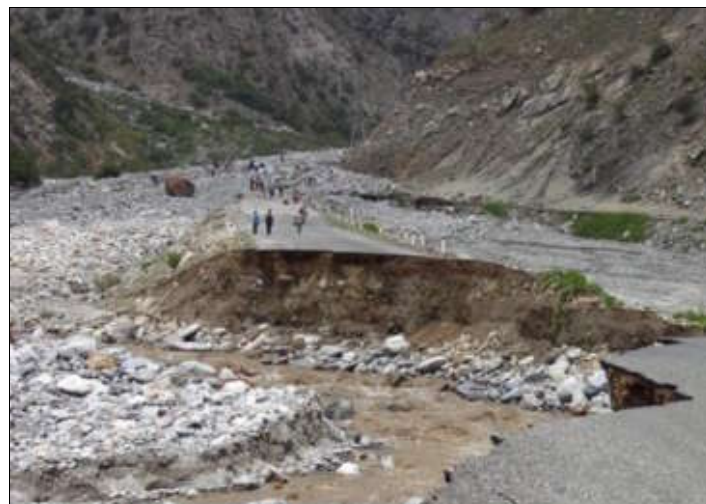
Figure 4: Varzob River, 40km north of Dushanbe, TJ. Torrential rains in mid-July 2004 caused severe flooding. The river banks were heavily eroded, the main road became impassable and water supplies in the capital city of Dushanbe were disrupted.
